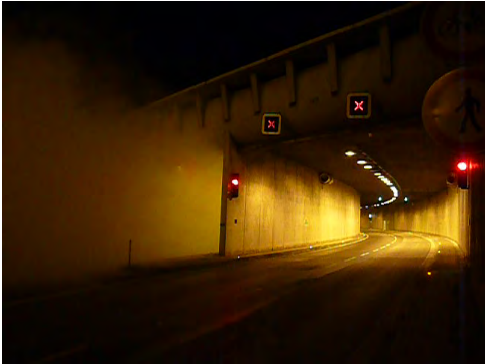
Figure 7. Portal of the Husovický tunnel during smoke test
