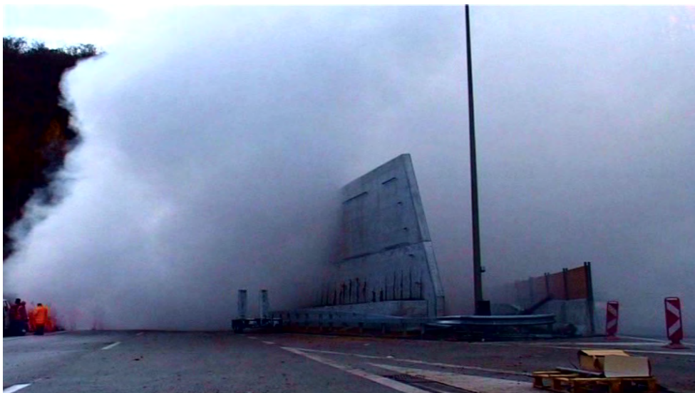
Figure 8. Spread of smoke over a dividing wall between tunnel tubes
