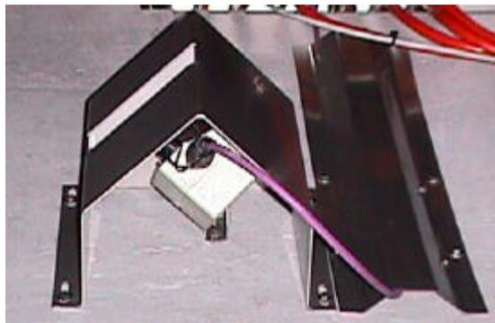
*Fig. 8 Ultrasonic anemometer in road tunnel*
